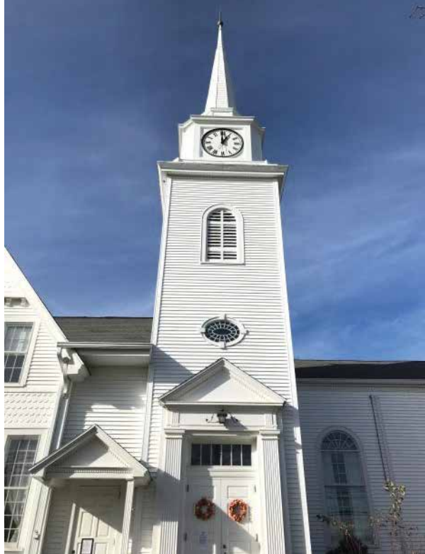
A capital campaign to upgrade the heating system and repair the steeple at the First Congregational Church of West Brookfield, UCC has been completed. SUBMITTED PHOTO
