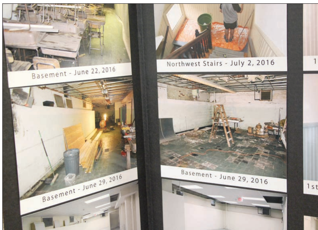
This display shows the work that went into renovating the school building.
